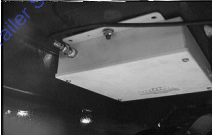
INSTALL ANTENNA CABLE
